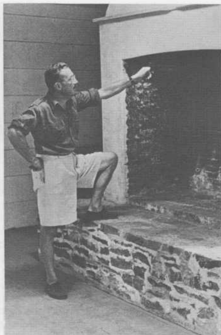
Col. Duncan Douglas inspects the massive stone fireplace in the second floor living quarters. The fireplace was recently rebuilt as part of D.O.T.'s restoration program.
