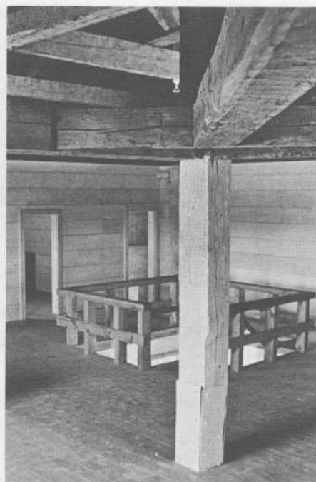
A view of the second floor, showing living quarters partitions, top of the staircase and the massive beams which support the ceiling.
