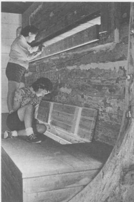
Helen peers through gun slots, while Kathryn sits on restored gunwalk and looks down to filled in moat. Boiling oil was poured through openings onto invaders who got close to blockhouse.
