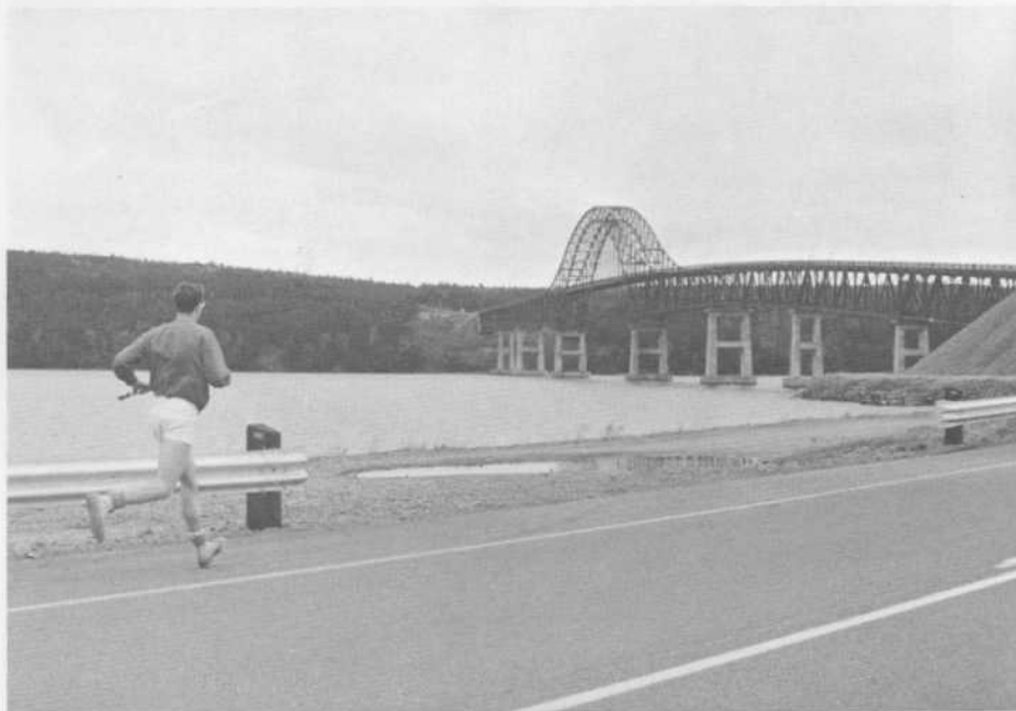
Cadet Tait approaches the Seal Island Bridge on the way back to the Canadian Coast Guard College.
