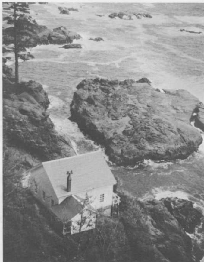
Pachena Point fog alarm building
