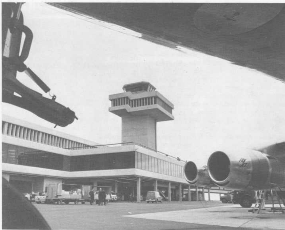
The unique control tower atop the new Vancouver International Airport passenger terminal presents a striking silhouette against the sky.
