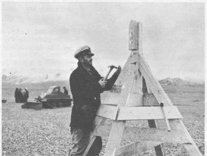
Ship's carpenter J. Ridgeway erecting a beacon at the northernmost section of Tanquary Fiord.
