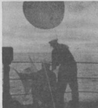
UPPER AIR-LEVEL OPERATIONS. On deck releasing a rawin-sonde balloon twice daily, average ascent, 55,000 ft. Radar office where course of rawin balloon is tracked by radar for upper wind information. Radio Officers W.M. Granger and G.M. Robertson at work.
